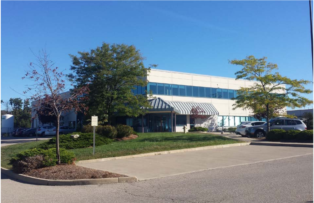
The new IDT Biologika building in Cambridge will be home to a state-of-the-art animal vaccine manufacturing hub serving North America.
